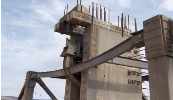
FIGURE 12 ‘TRADITIONAL’ MOMENT CONNECTION: COMPLETE COLUMN DEMISE AND SEVERE GLOBAL DEFORMATION OF TEST ARTICLE WITHOUT COMPROMISING THE CONNECTION, ABSENT FLOOR GRAVITY LOADS.
